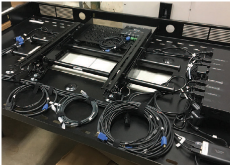
Pre-built in our assembly facility
